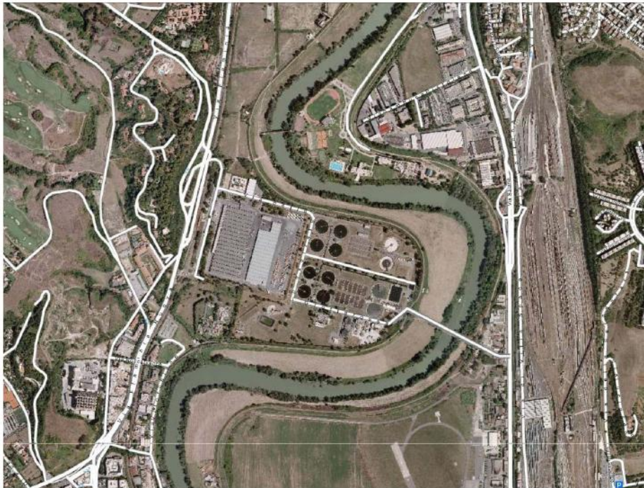
Fig. 8 .View of Roma Nord treatment plant
